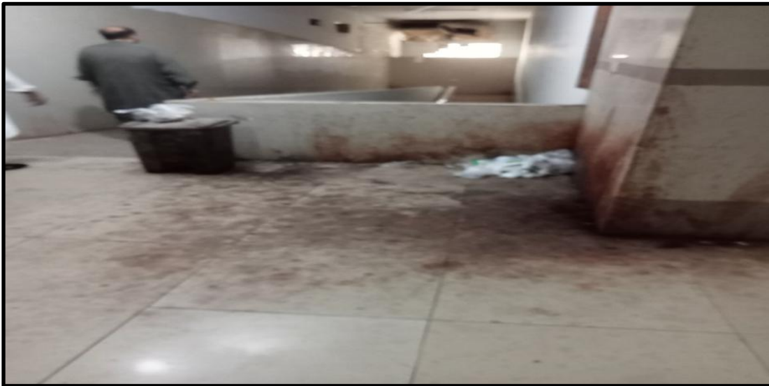
(Janitorial Condition of Abbasi Shaheed Hospital)
